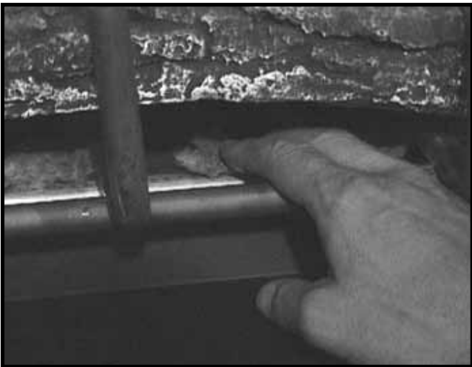
Figure 14.5 Placing the Rockwool
