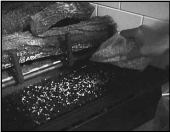
Figure 14.4 Placing the Vermiculite
