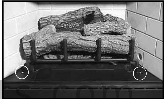
Figure 14.6 Remove Two Screws Holding Front Grate/Log Assy.
