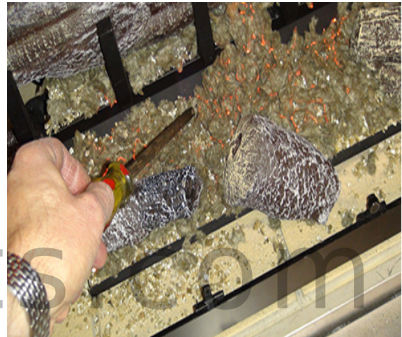
Figure 9- Adjusting of Flame Pattern
