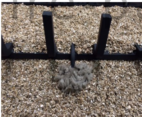
Figure 8b- Packing rock wool around the carry over tube
