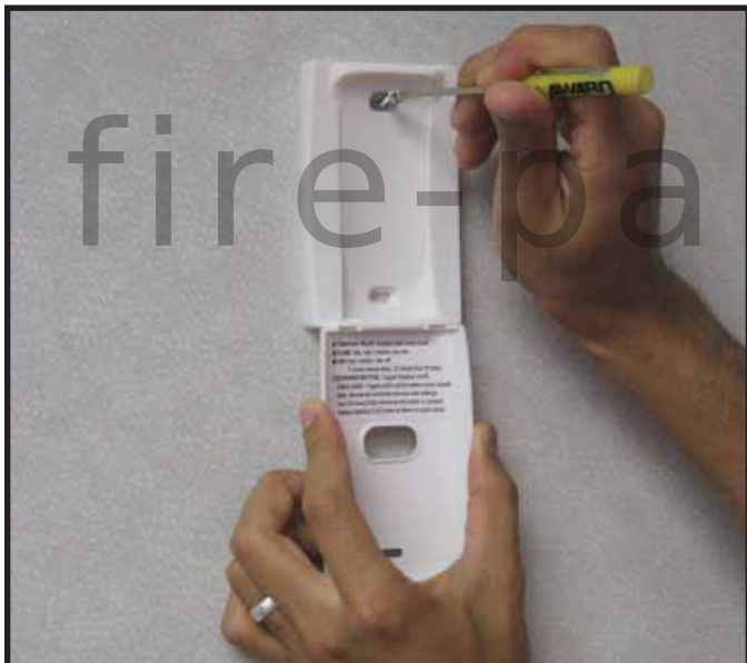
Figure 1. Mounting Remote Control Housing
