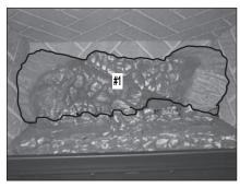
Figure 8.23 Place rear log onto the two locating pins located on the rear log shelf in the back of the firebox.
