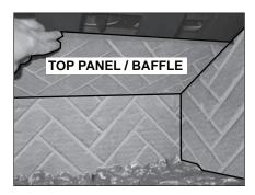
Figure 8.18 Install top panel/baffle. If rear venting, set the damper prior to installing top panel/baffle. Holding panel at an angle, place one end on top of side panel and lift other end into place. Move left or right until centered.
