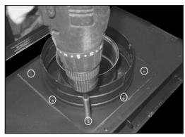
**Figure 8.2** Remove vent pipe adapter and gasket by removing 8 screws. Save the screws. (If gasket breaks, apply high-temp sealant to bottom of adapter before installing as shown in Figure 8.8.)
