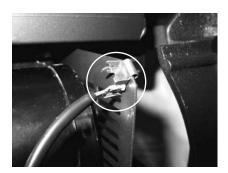
Figure 8.28 Attach grounding clip supplied with the kit to the blower housing. Attach ground wire to grounding clip.
