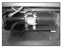
Figure 8.27 From the rear of the appliance, slide the blower into the blower housing with the magnetic strips down. The blower openings should be at the front.
