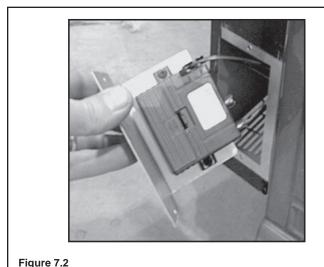
The ignitor is located on a plate attached to the side of the appliance using two #8 Phillips head screws. To access the ignitor, remove the two screws securing the plate to the side of the appliance and slide the plate out.
