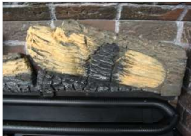
Log "B" installed correctly
