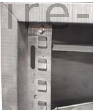
LOUVRE SNAPPED INTO PLACE
