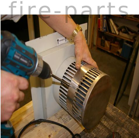
Take the top half of the new stainless steel termination and slide it over the body of the old termination to the halfway point of the old termination. Once the new half stainless steel termination is in place screw down with three tec (1/4") screws.
