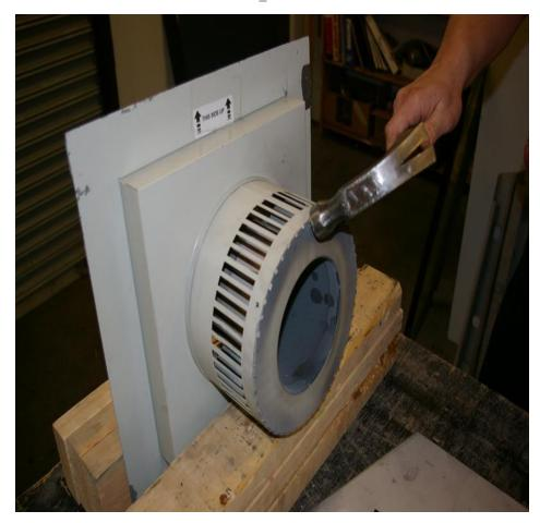
After removing the top half of the old termination, hammer down the end pieces of metal that may be protruding from the termination. This will allow for a nice neat finish.
